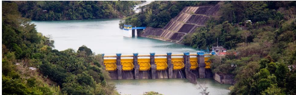
Ipo Dam (MWSS / MANILA BULLETIN)
