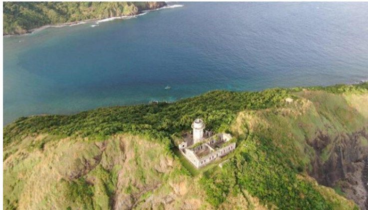
An aerial photograph of the historic lighthouse on Palaui Island
