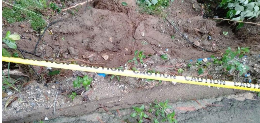
Landslide in Cebu City. | Photo Courtesy of Cebu City PIO
