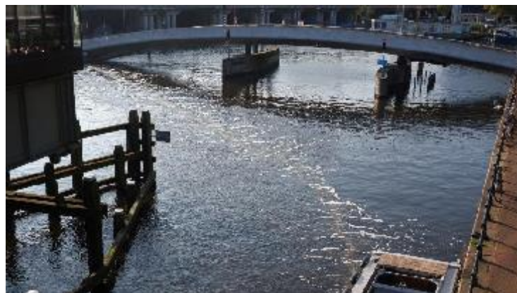
Bubbles guide trash to the catchment system, bottom right.
