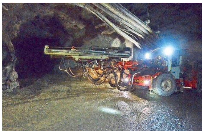
A jumbo drill travelling inside the exploration decline.
