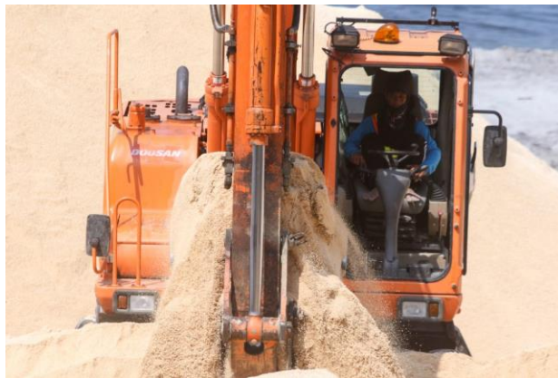
Workers pile the “white sand” to be laid on Manila bay. (Jansen Romero / MANILA BULLETIN)
