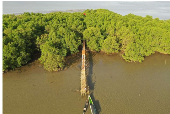
Aerial view of the Sasmuan Bangkung Malapad Critical Habitat and Ecotourism Area showing its receiving area and wooden boardwalk.
