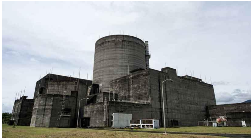
Bataan Nuclear Power Plant -- BW FILE PHOTO
