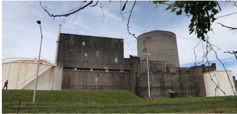
Bataan Nuclear Power Plant. PHOTO BY RENE H. DILAN
