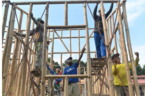
Workers make use of bamboo as construction material.
