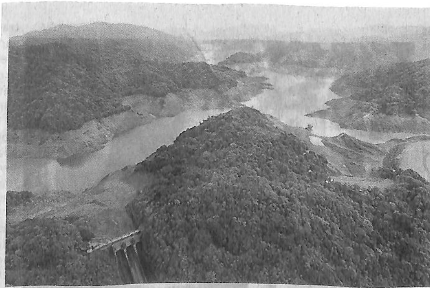
Angat Dam supplies Metro Manila and nearby provinces with water
