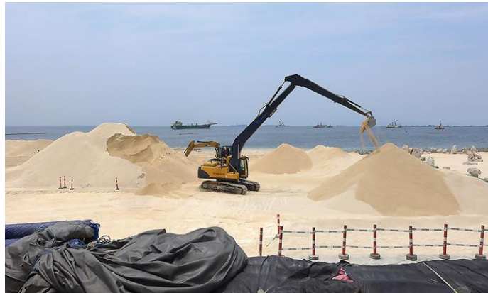
In this April 15, 2021, file photo, heavy equipment dump dolomite sand over a portion of Manila Bay along Roxas Boulevard in Manila to create an artificial beach.
