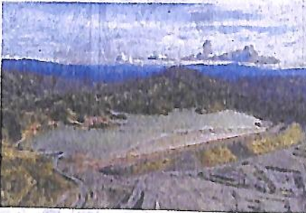
The Tailings Storage Facility has a treatment capacity of 1,980 cubic meters per hour
