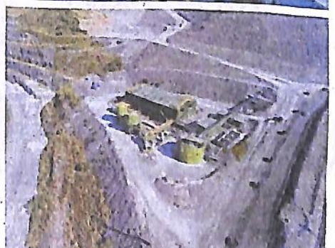
The Paste Backfill Plant produces a monthly 50,000 cubic meters of paste.
