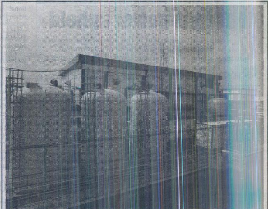
This NEW WATER Treatment Plant in Parañaque is Maynilad's first facility that converts "used water" to water that meets the Philippine National Standards for Drinking Water. Equipped with treatment technology from Israel—a world leader in water innovation—this facility can produce 10 million liters of potable water per day. It is the first "direct potable water reuse" application in Asia.
