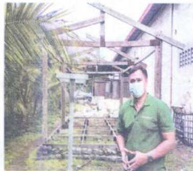
Envirohome, a 28-sqm house made with recycled plastic waste, where 95 percent of the materials are made with soft plastic waste.
