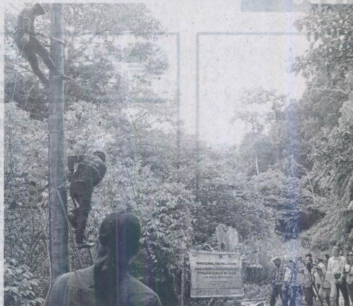
PROTECTING EAGLES Linemen of the Cotabato Electric Cooperative install on March 24 the insulated wire at the electric post where an eaglet was electrocuted in 2018. —PHOTO COURTESY OF PHILIPPINE EAGLE FOUNDATION
