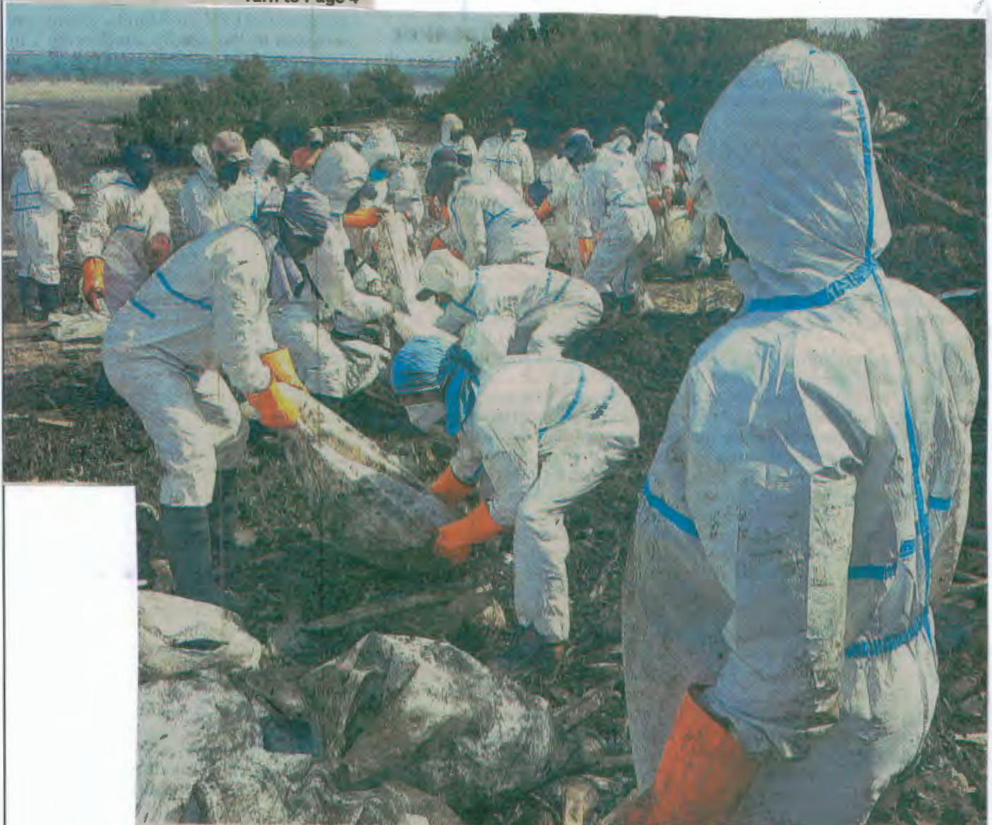
Responders from Semirara Mining and Power Corp. clean up oil spill from the sunken tanker in Oriental Mindoro on Monday. SMPC partnered with the Department of Energy, Philippine Coast Guard, Office of Civil Defense and Department of Health.
