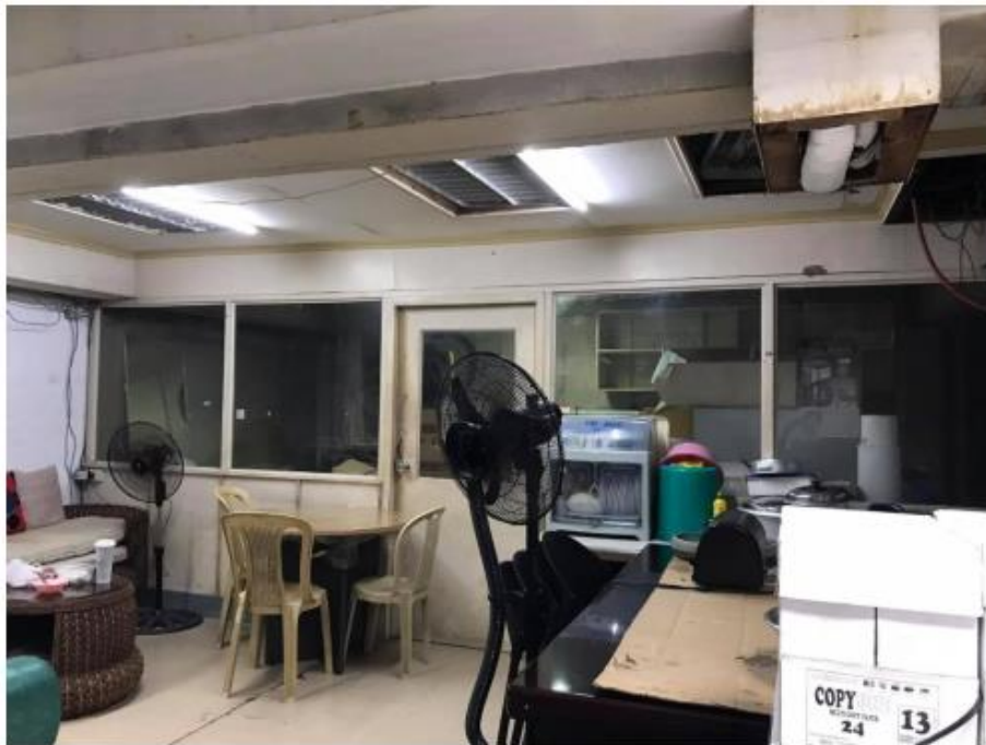
PIC 2: PICTURE TAKEN OPPOSITE SIDE OF THE ENTRY
