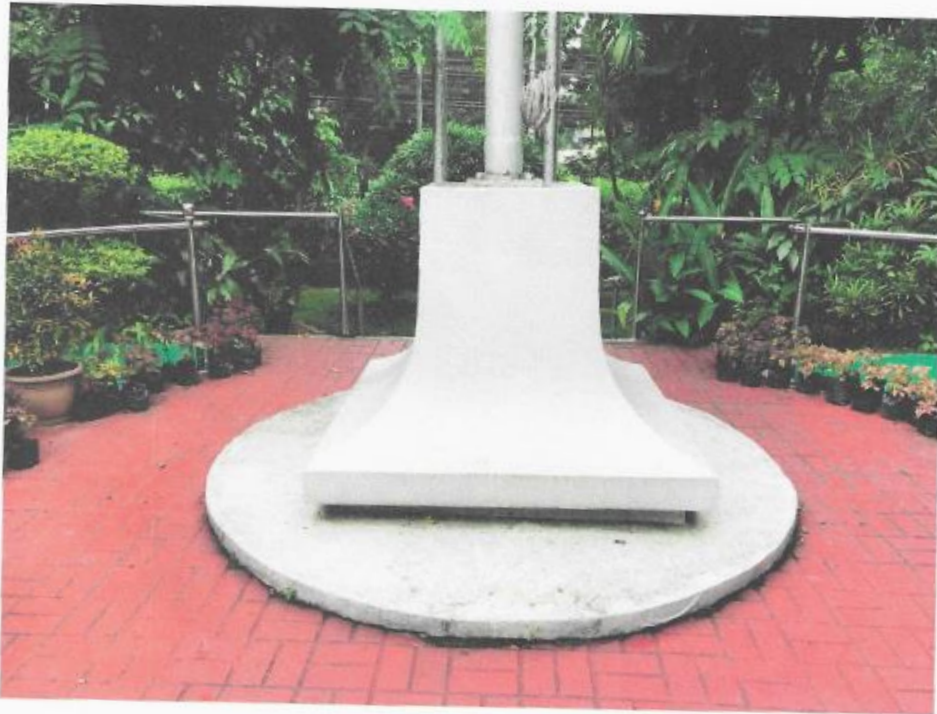
PIC 2: EXISTING PEDESTAL OF THE MIDDLE POLE
