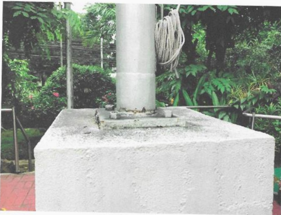
PIC 3: EXISTCONNECTION BETWEEN THE POLE AND THE PEDESTAL
