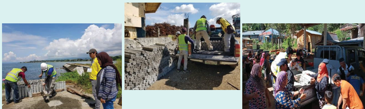
Figure 22.3 Photos during fabrication, hauling and establishment of monuments
