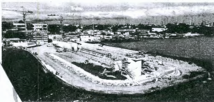
Water treatment plant being built in Poblacion, Muntinlupa.
