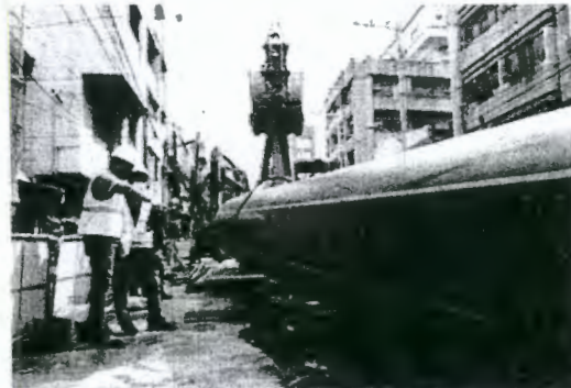
Installing new sewer pipeline.
