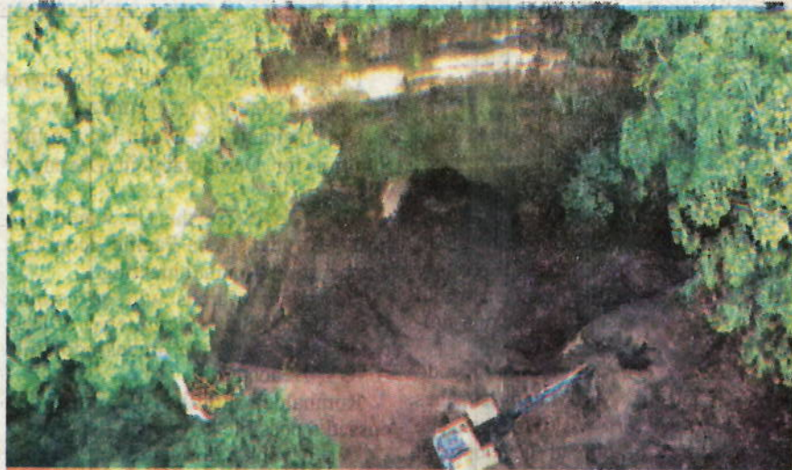
CAVERNOUS. The 200-meter wide and 30-meter deep tunnel discovered inside the New Bilibid Prison leads to a river and was dug below a swimming pool. Screengrab from ABS-CBN's drone footage
